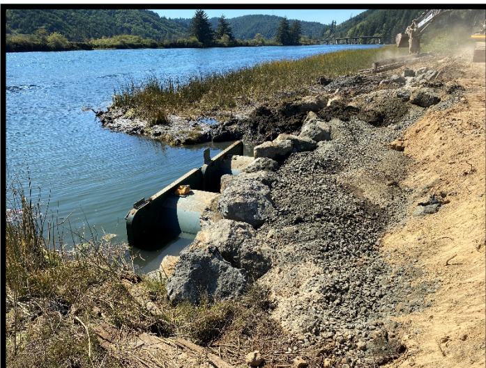
September 2023 – Set of tide gates in process of being installed.
