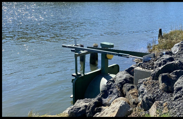
September 2023 – Single tide gate and culvert installation.
