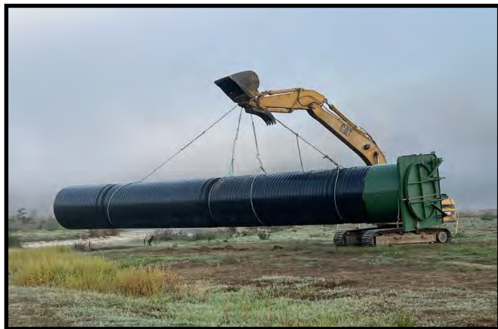
September 2023 – One tide gate & culvert being moved to the installation location.
