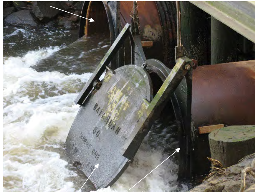
Tide Gate & Culvert in Good Condition
