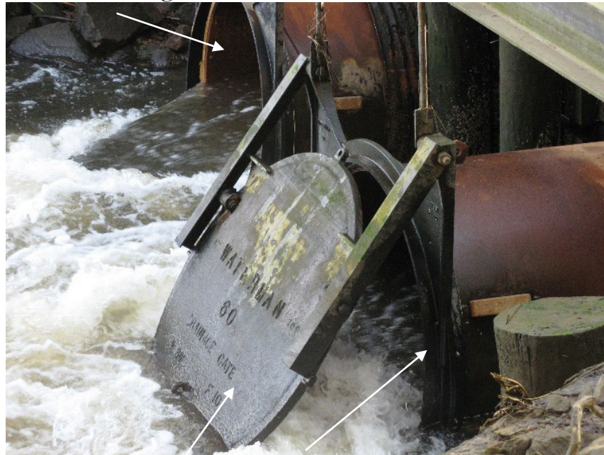
Tide Gate & Culvert in Good Condition
